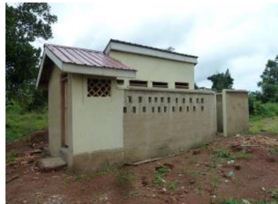
The toilets are of traditional design and do not have the venting which is characteristic of the newer Blair-VIP design. The original classroom block has had the floor relaid and the walls plastered and painted. One of the rooms is shown on the front page of this report where the students are dancing and singing.
