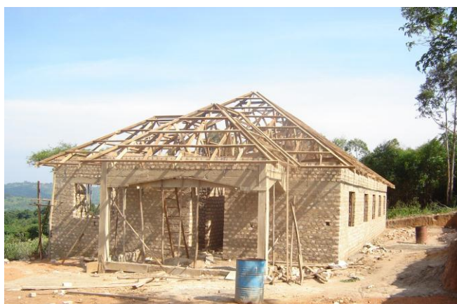
Work on Girls' Dormitory at Isaac Newton School
